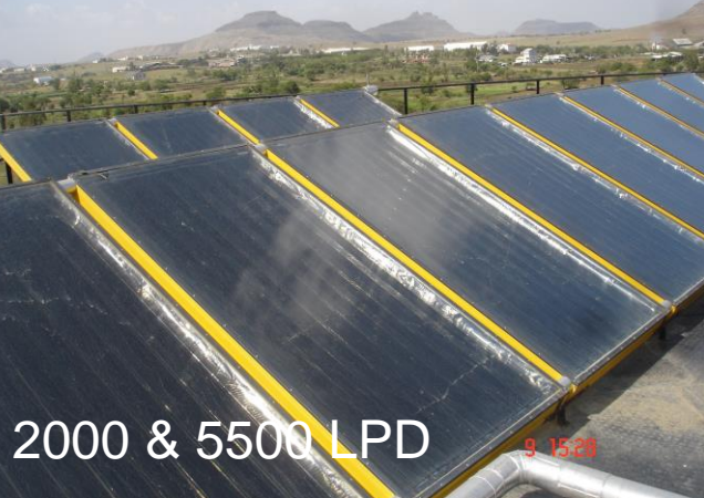
Solar water heaters
