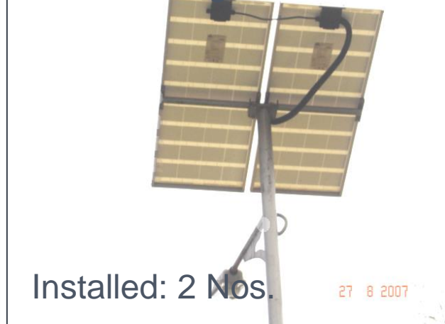
Solar street light
