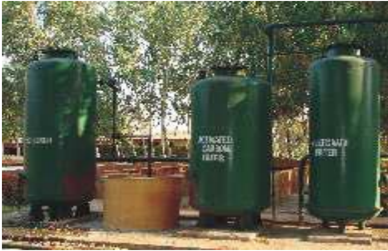
Waste water treatment plant
